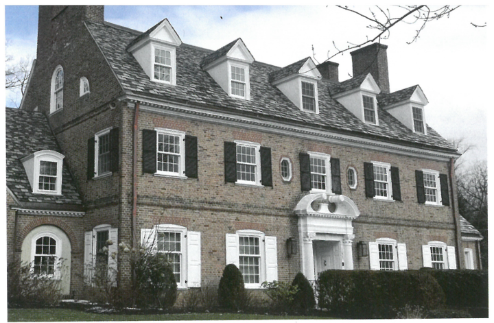
The Anchorage, a private residence, is a gracious example of Colonial Revival architectural style, drawing specifically from original Georgian prototypes. The elaborate front entry features a prominent broken pediment. Dentils are seen at the cornice and in the front entry structure.
