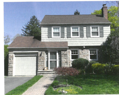
This 1940s interpretation of the now includes a one-story overhang, the attached garage, and masonry façade. The sidelights on either side of the front door are true to classic Colonial Revival
