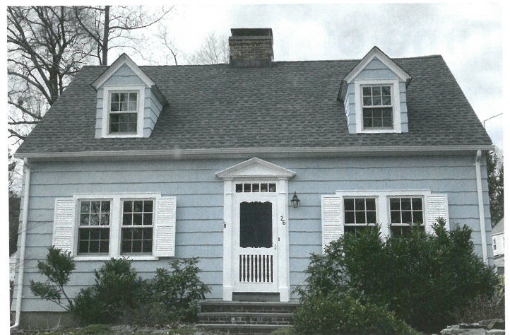
This Cape Cod is true to its Colonial Revival style, with dormers, paired windows, and a central chimney. The pedimented front door even features a transom window reminiscent of a fanlight.
