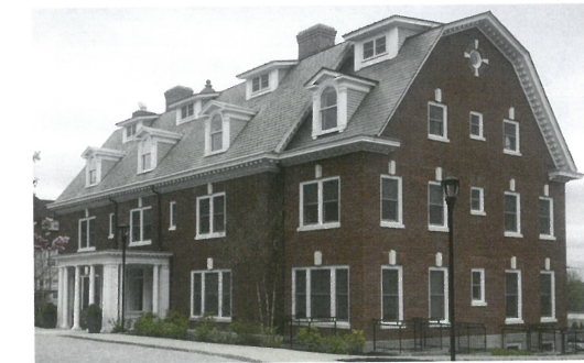
The gambrel roof of The George places it in the Dutch Colonial Revival subtype. The elaborate front portico supported by columns, dentils at the cornice line, windows groupings, and dormers with pronounced pediments are classic revival elements.
