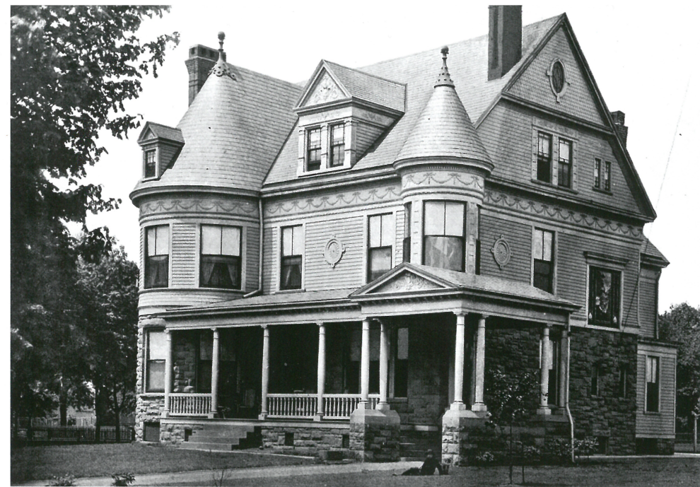
This home on Park Street has not only a tower on the left side of the front porch but also a turret on the right corner of the front façade. The turret does not extend below the covered front porch roof. Both the turret and the tower have a conical roof and feature decorative finials. There is also a narrow Porte Cochere at the right end of the front porch.
