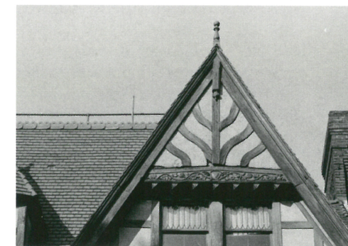
This photo shows a finial, bargeboard, and a half-timber gable. The bargeboard/vergeboard is plain on either eave at the sloped portion but is a carved decorative board above the window.
