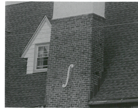
Anchor Plate/Tie Rod/Patress Plate: The “S” or “star” that you might see on the face of a chimney or randomly placed on a brick wall. Typically seen in older construction, a metal tie rod with an anchor plate used to stabilize or “tie” the brick exterior or tall brick chimney to the inte-
