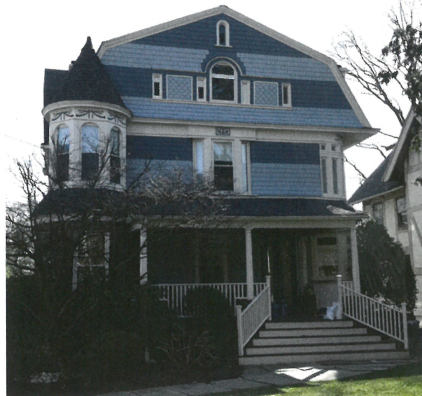
A Palladian window below the gable peak, is set among varied wall surface materials in contrasting colors, a roof gable that extends beyond the curved window below it on the right, and a turret on the left with decorative swag embellishment
