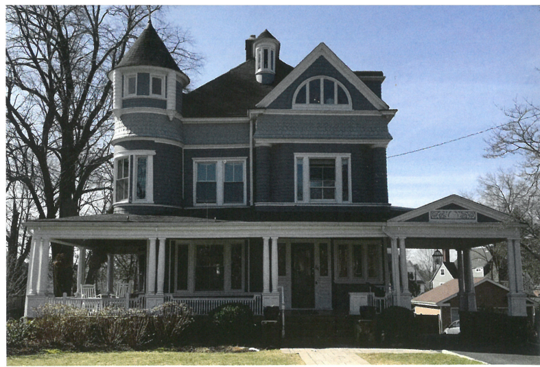
The paired, classic columns supporting the wide porch are common Queen Anne features, as is the front-corner turret, contrasting wall surface materials; and other unique ornamentation.
