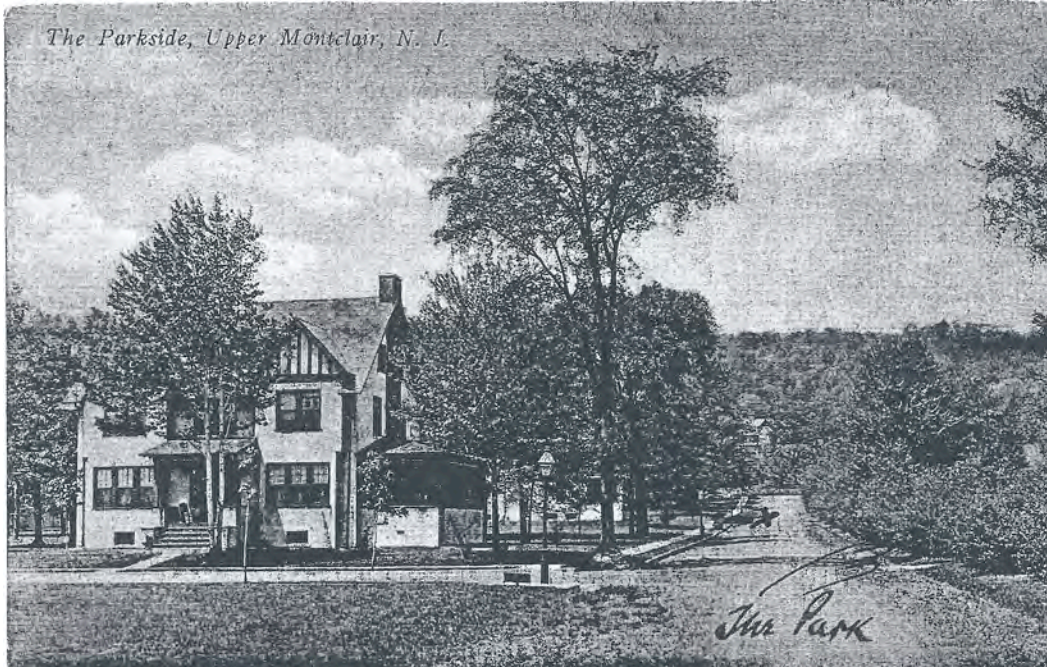
Figure 4: 130 Edgemont Avenue, with a view of The Parkside, looking west. Anderson Park is to the right. Undated.
